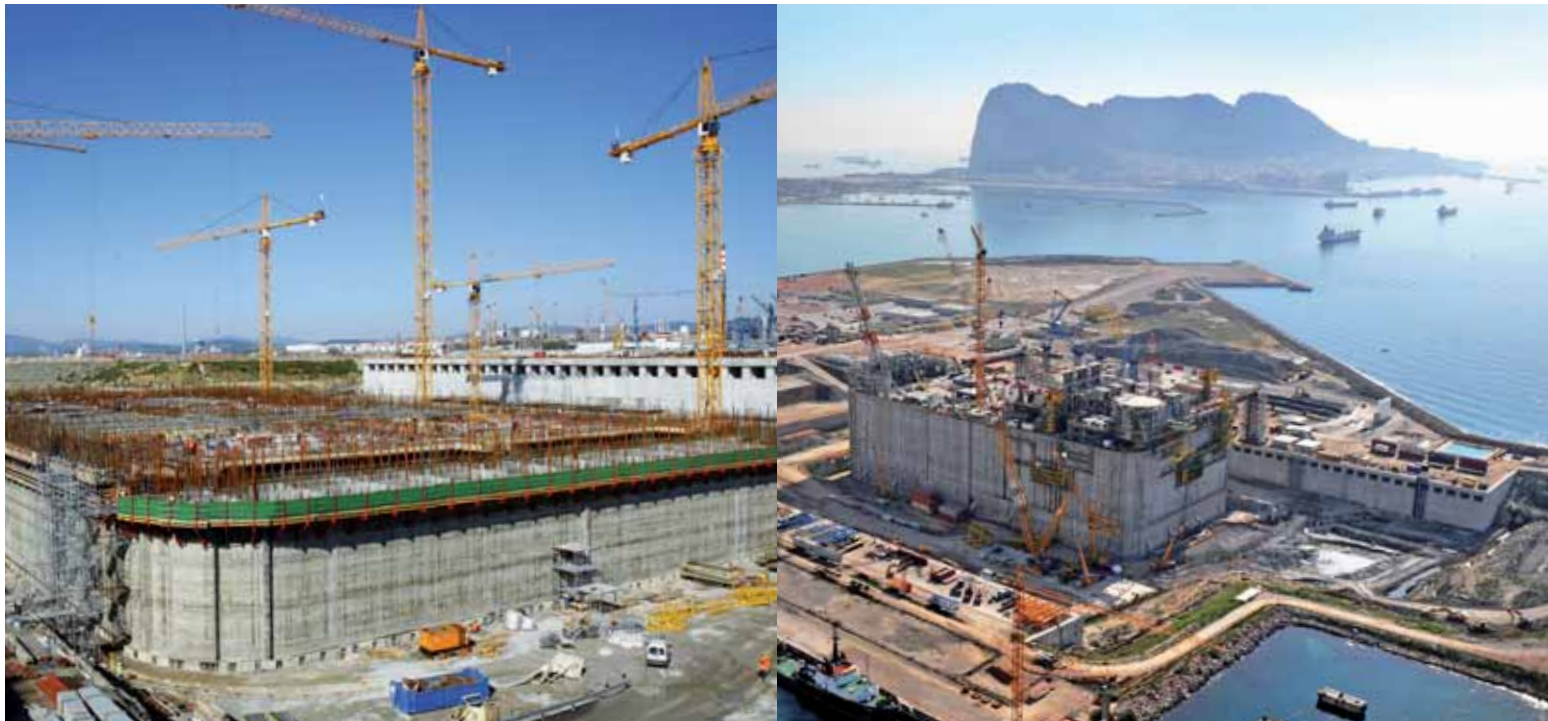
The Adriatic LNG regasification terminal was built at a shipyard in Algeciras (Spain), towed to the Adriatic Sea and positioned offshore Porto Viro (Rovigo). The event held on September 20, 2008 to celebrate its arrival was attended by Silvio Berlusconi, Italy's Prime Minister.
