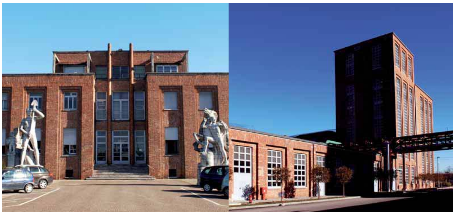
The new Torviscosa (UD) power plant is being built next to a landmark Snia facility, providing a perfect architectural bridge between past and present.
