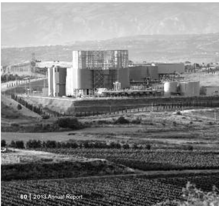
View of the Altomonte (CS) combined-cycle thermoelectric power plant.
