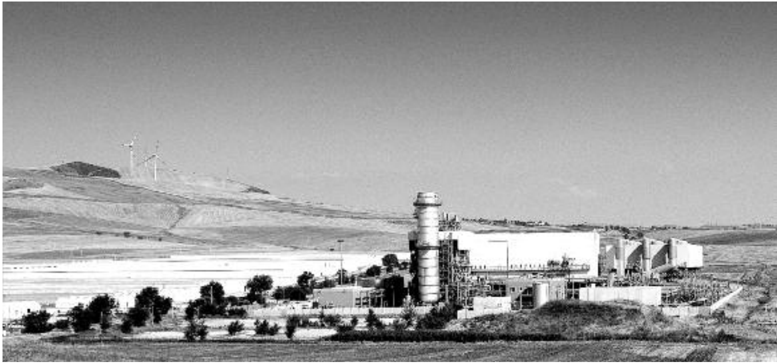
A bird's-eye view of the Candela (FG) thermoelectric power plant.
