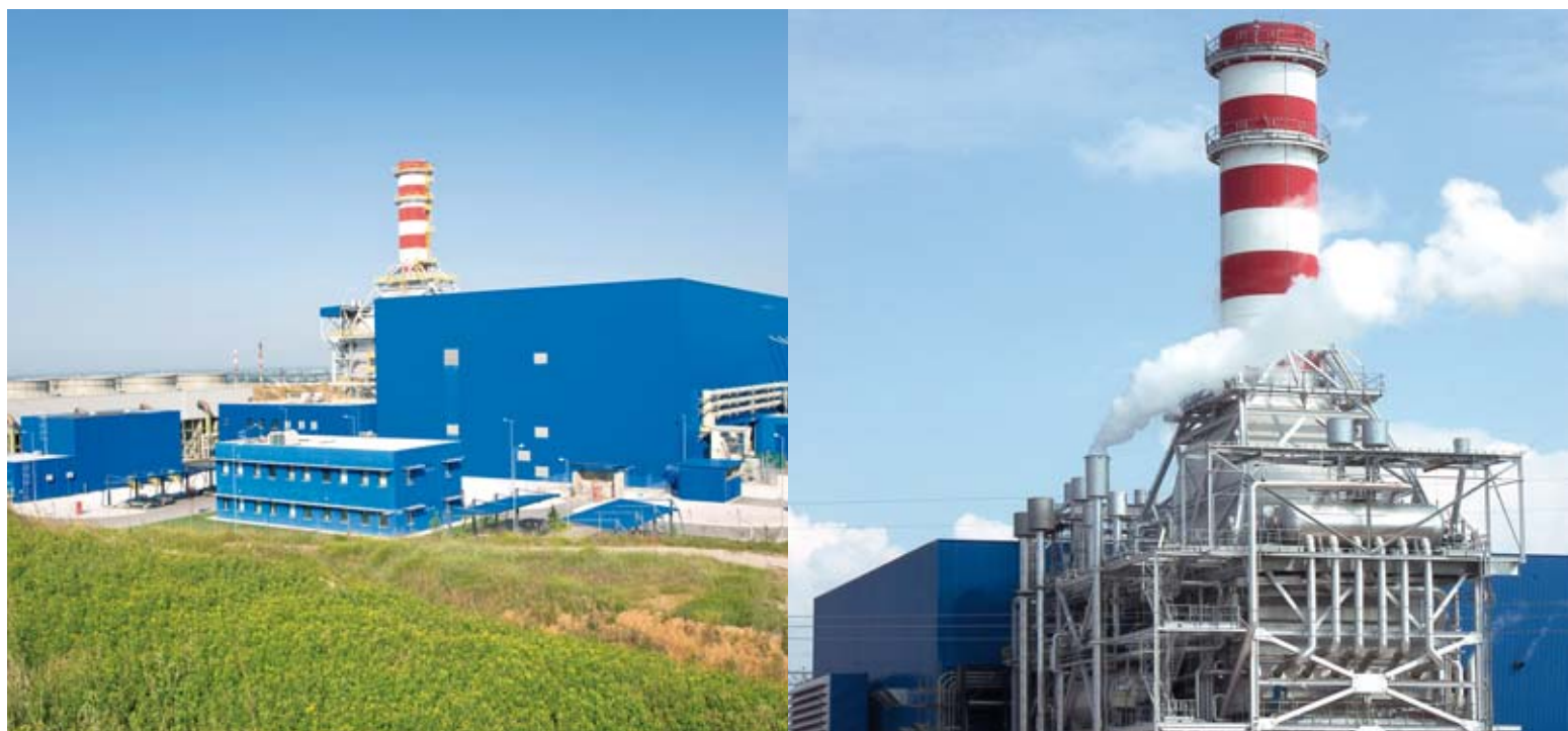
In Greece, the Elpedison joint venture operates a 390-MW thermoelectric power plant in Thessaloniki and a new 420-MW power plant in Thisvi.
